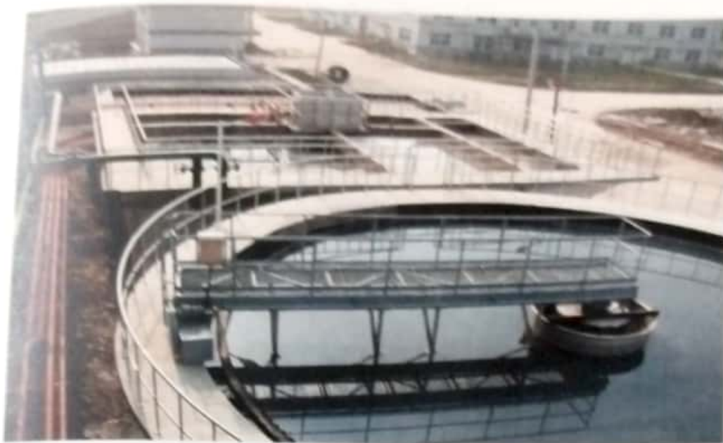
Fig. 3.2 Sedimentation Tank
